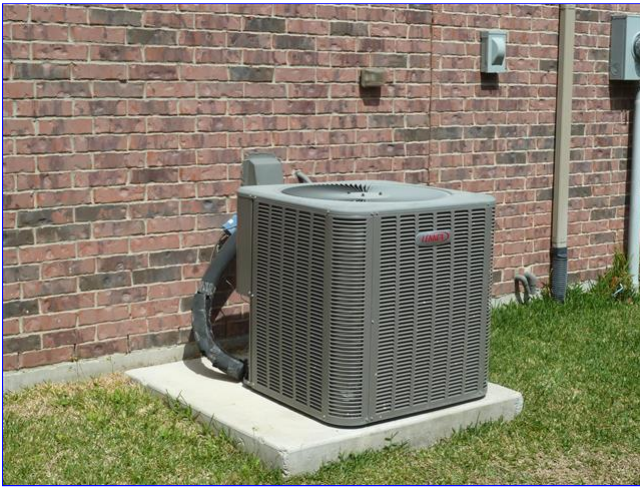
B. Item 1(Picture) Condensing unit
