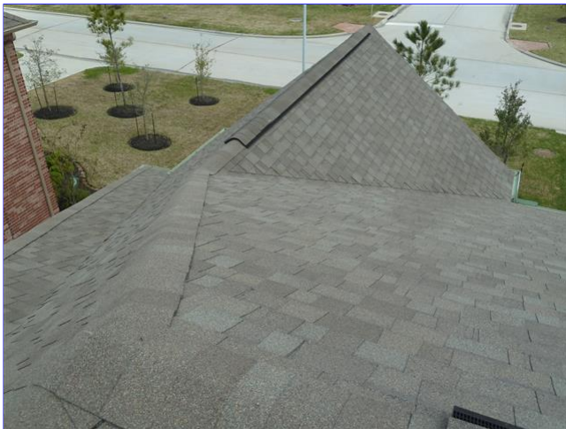
C. Item 2(Picture) Roofing materials and ridge vent.
