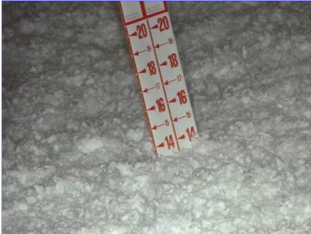
D. Item 1(Picture) Blown in attic insulation.
