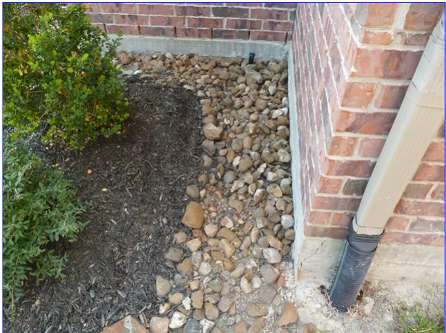
B. Item 1(Picture) Adequate slope, grade, and gutters.
